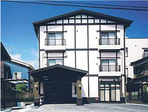
Photo 6 Exterior of Jizodo
